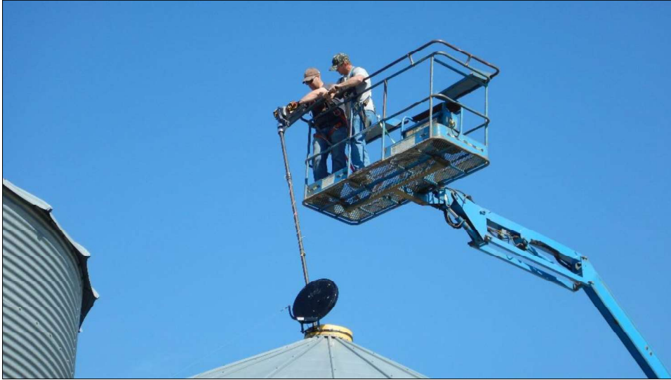
Figure 3. Probe installation process.
